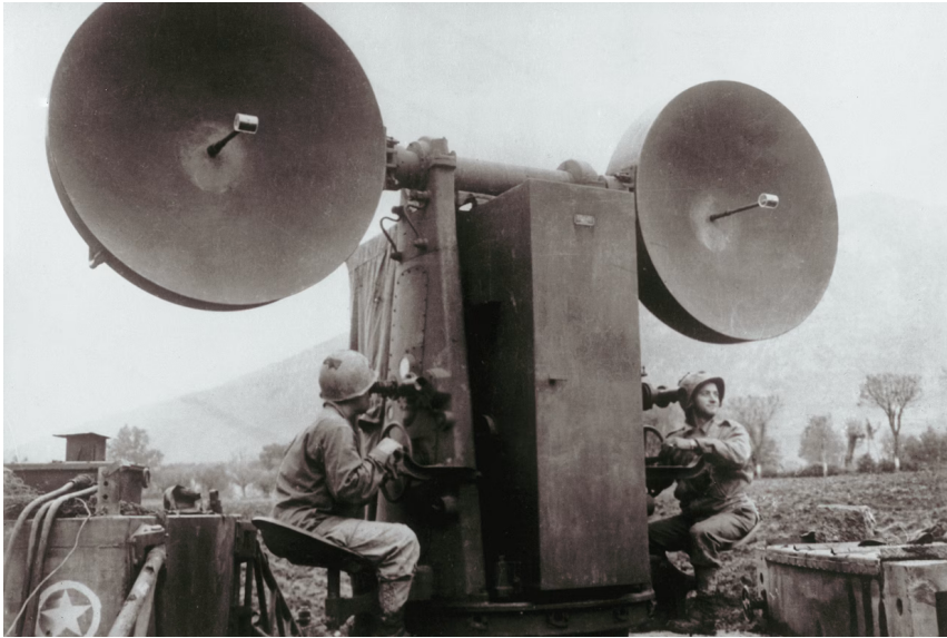
An American radar system used to direct anti-aircraft guns in World War II. PHOTO: BOYER/GETTY IMAGES
